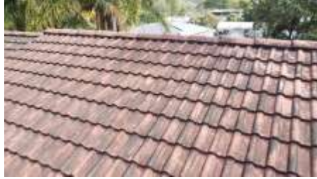
Roof photos taken by Drone
