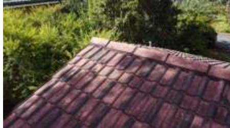
Roof photos taken by Drone
