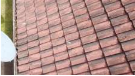
Roof photos taken by Drone
