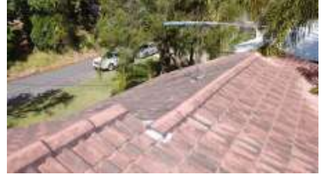
Roof photos taken by Drone
