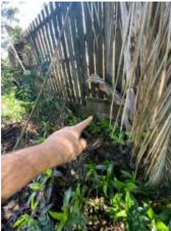
Concrete block boundary walls leaning to parts, recommend engage a Builder to rectify.
