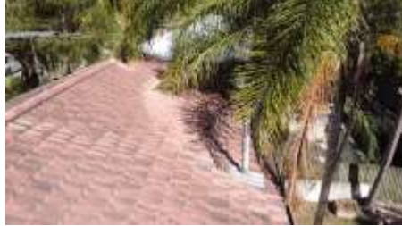
Roof photos taken by Drone
