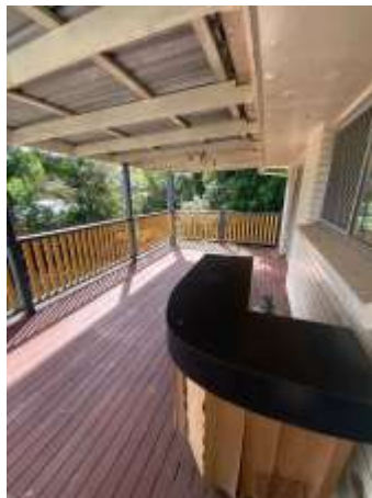
Showing General photos
