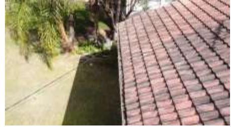
Roof photos taken by Drone
