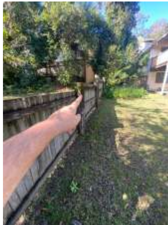
Concrete block boundary walls leaning to parts, recommend engage a Builder to rectify.
