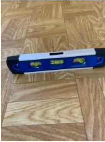
Undulating/uneven floors - recommend engaging a Builder to assess appropriate method of rectification to prevent further deterioration.
