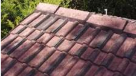
Roof photos taken by Drone
