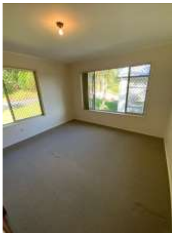
Termite damage noted to the Wall Skirting in Bedroom 2, Highly recommend engage a Builder for further investigation to determine the extent of damage and repair proposals.
