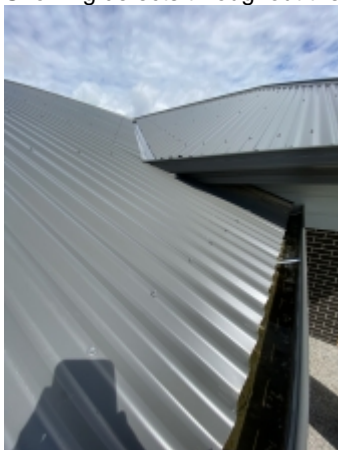
Showing general photos of the property
