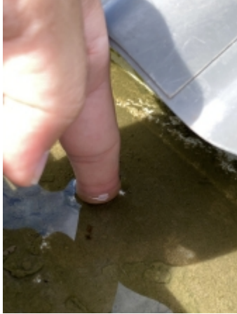
Showing defects throughout the property
