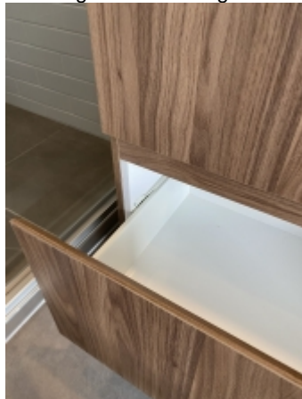
Showing defects throughout the property
