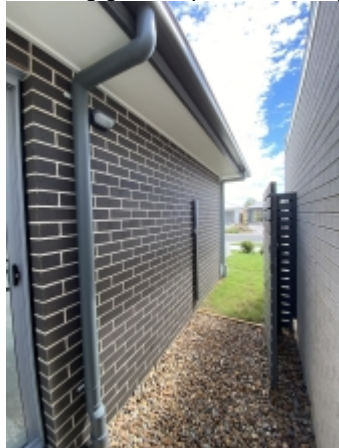
Showing general photos of the property
