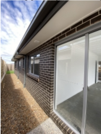
Showing general photos of the property
